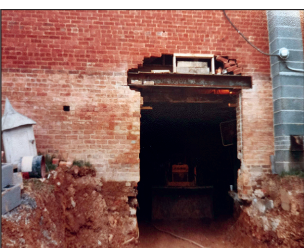
Adding a basement
